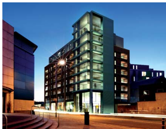
New flats in Hardwicks Way
